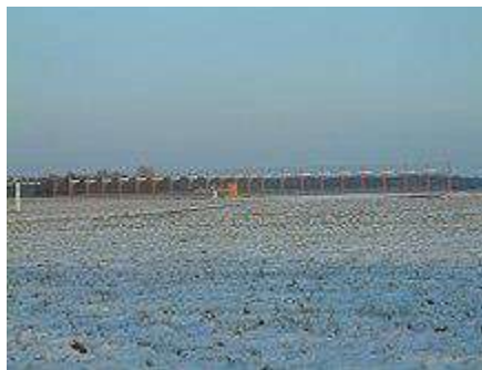
The localizer station for runway
