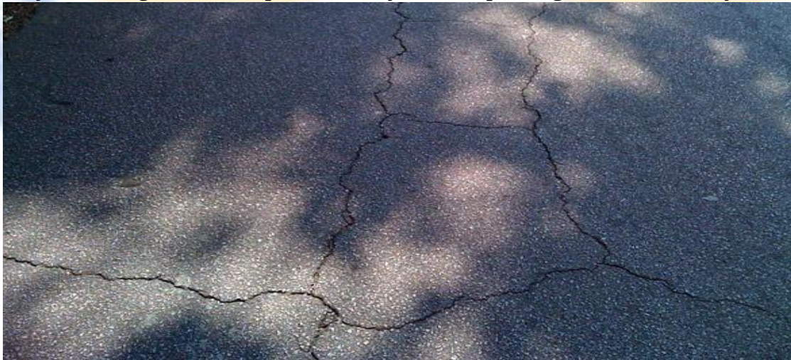
Fig.BlockCracking
