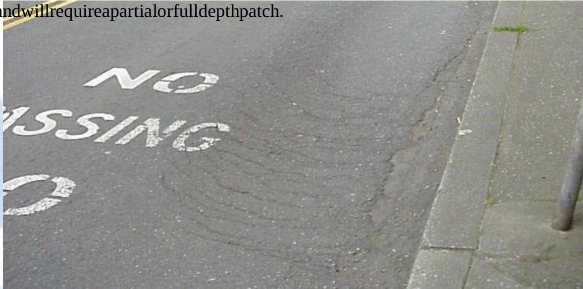
Fig.SlippageCracks
