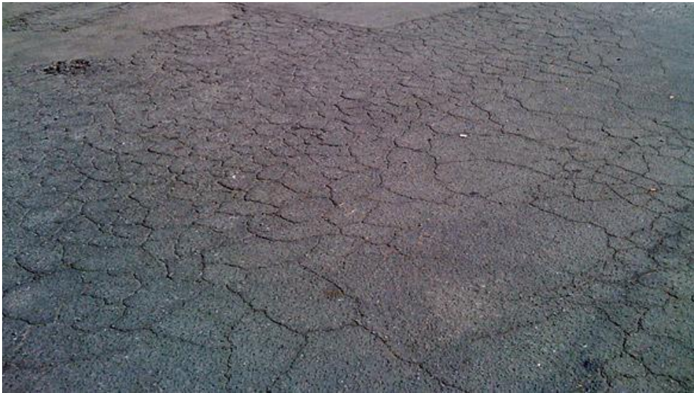
Fig.AlligatorCracking
