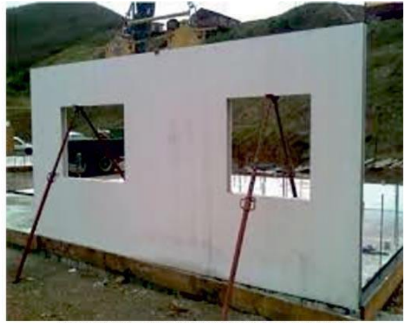
Figure 10: Glass fibre reinforced gypsum panel system
