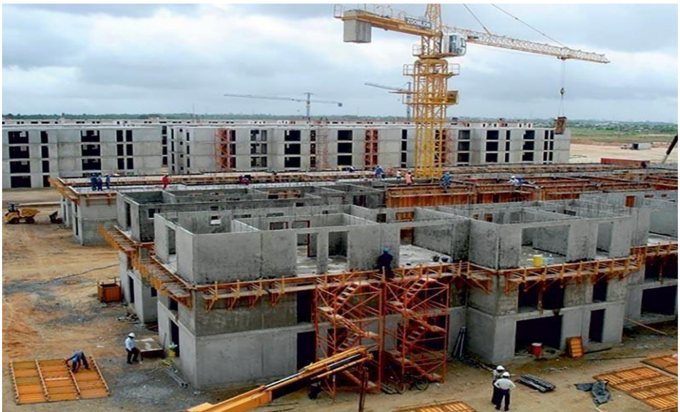
Figure4:Kayson'sformworksystem construction
