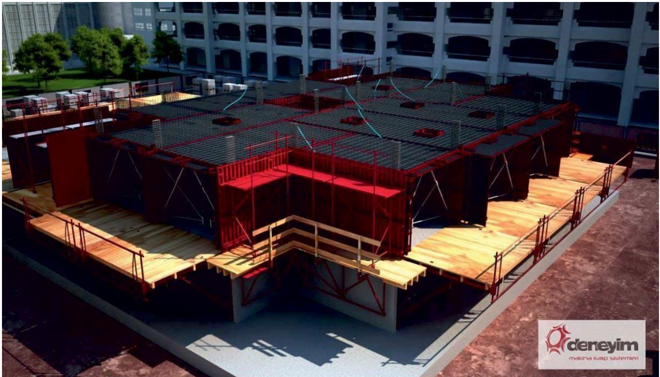
Figure3:Cellularconstructionusingmodulartunnel
