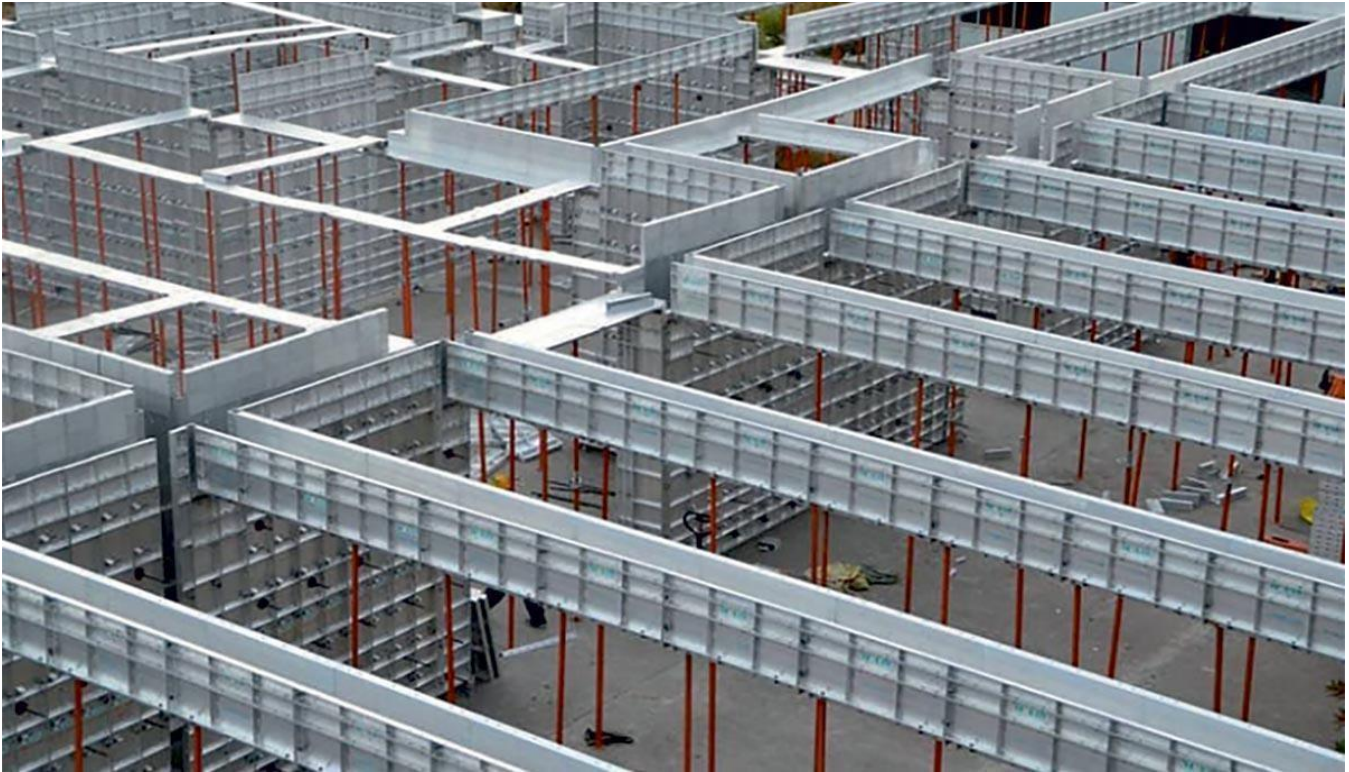
Figure2: Monolithic construction by aluminium plastics
