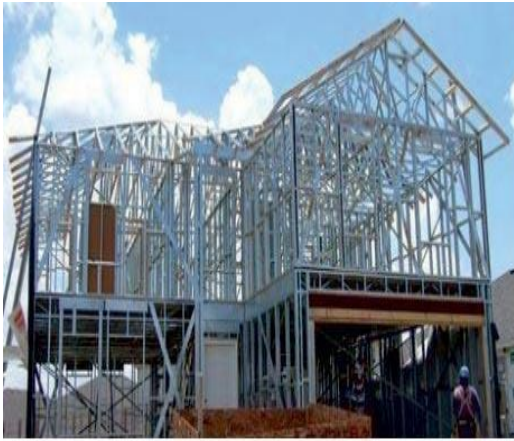
Figure 11: Light Gauge Steel Structural Systems Pod
