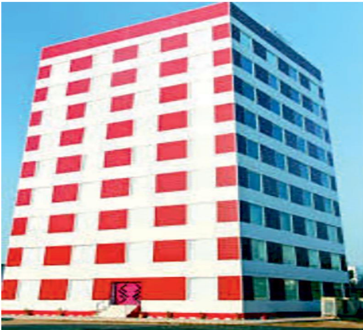
Figure 16: Factory made fast track modular building system
