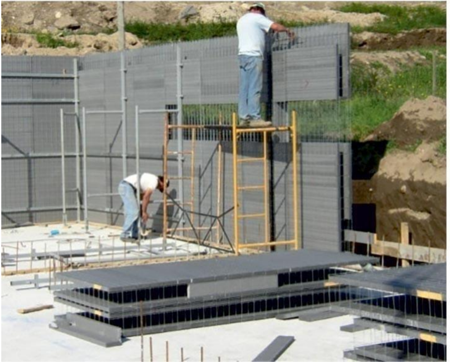
Figure5:ConstructionofawallwithSismoTechnology
