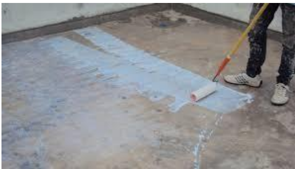
Fig.1. Application of Latex Bonding Agent
