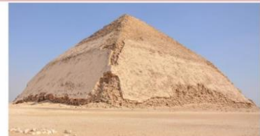
BENT PYRAMID: Unique amongst the ancient Egyptian pyramids is the aptly-named Bent Pyramid, the slope of which changes roughly two thirds of the way up. The lower part of the pyramid is angled inward at roughly 54 degrees, then at 49 metres above the base it flattens out abruptly to 43 degrees, creating a distinctively bent shape.
