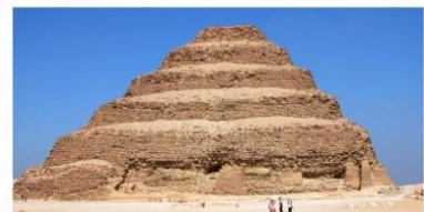
STEPPED PYRAMID: Stacking mastabas on top of one another and building in stone as opposed to the traditional mud-clay of other mastabas (for the king of the Third Dynasty of Egypt).
